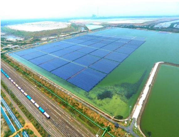
Ramagundam Floating Solar Panels
