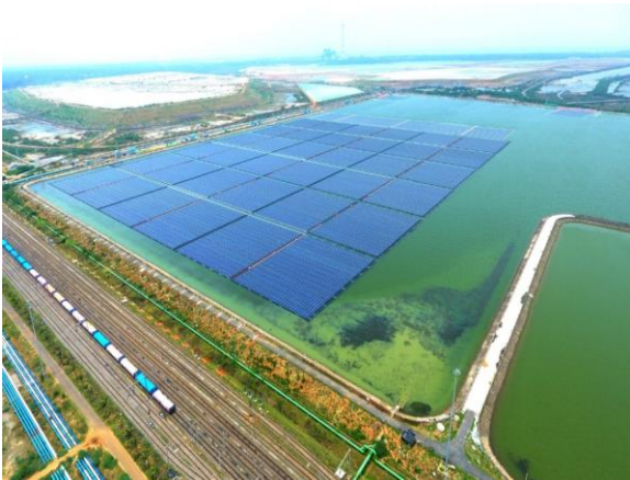
Ramagundam Floating Solar Panels
